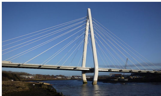
Northern Spire Bridge, Sunderland UK
