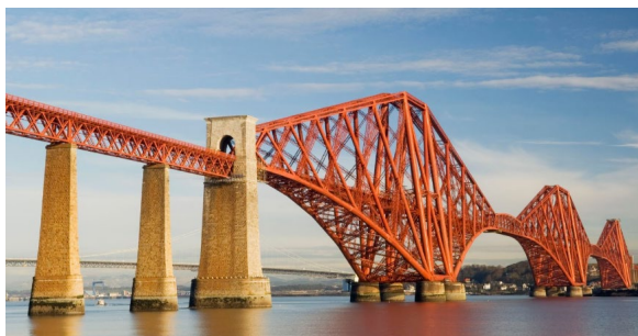
Forth Rail Bridge, Edinburgh UK
