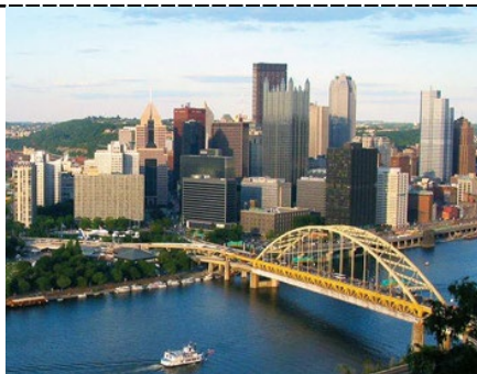
Fort Pitt Bridge, Pittsburgh USA
