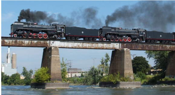
Iowa River Bridge, Iowa USA
